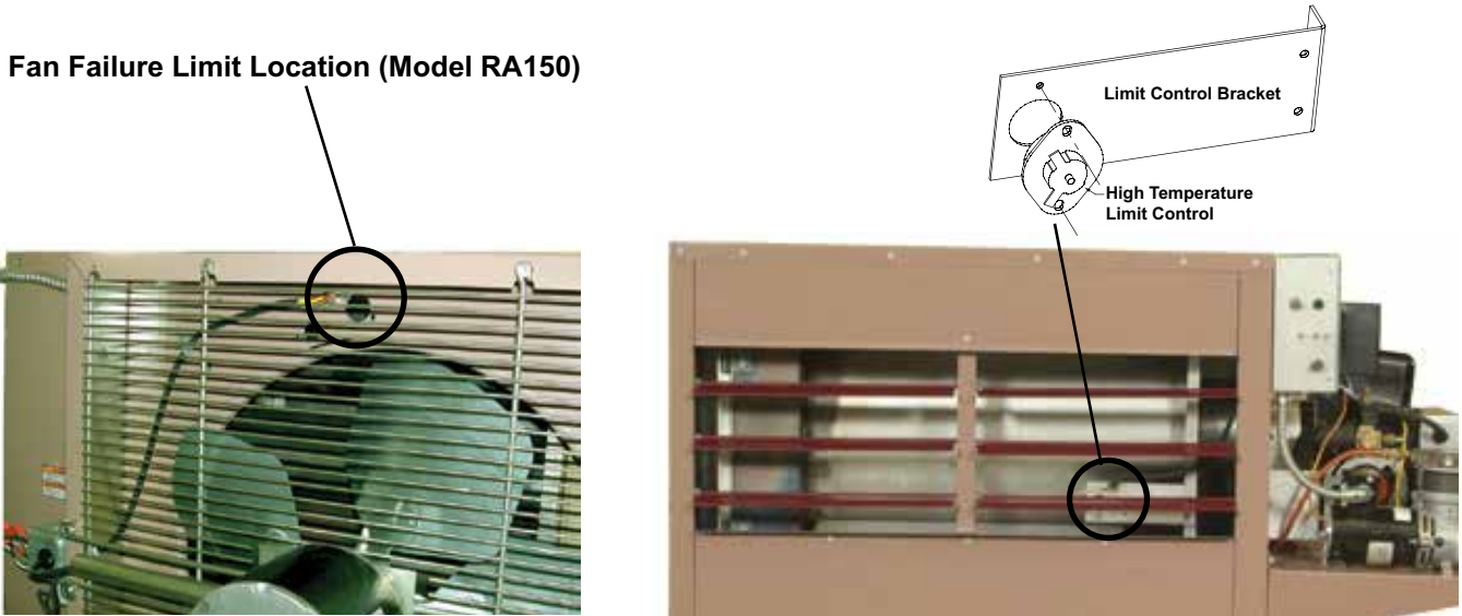
Figure 11. Limit and Fan/Blower Control Components and Access Location—Model RA/RAD, Unit Sizes 150 and 250 (Refer to Table 11 and Table 12 )
