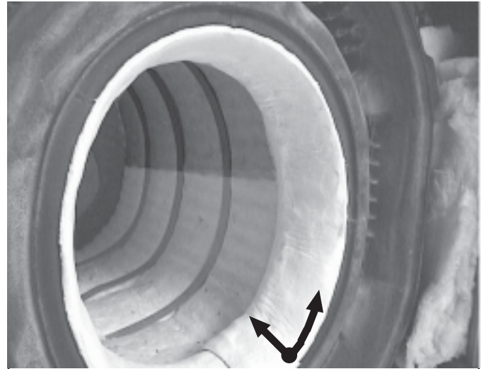
FIGURE 8 - Mold the liner starting at the bottom and working from the front toward the back. Keep the outer edge even with the opening; mold any excess at the bottom half over the edge of the chamber liner.
