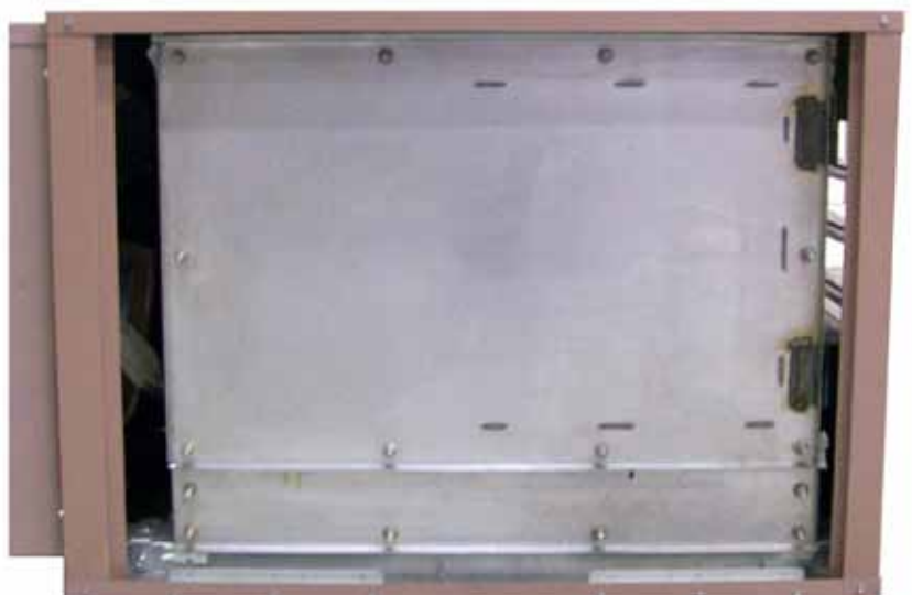
View of Hinged Inner Door with the Outer Access Door Removed
