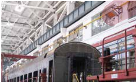
Model RIH - High Intensity Radiant Heater in a Train Station
