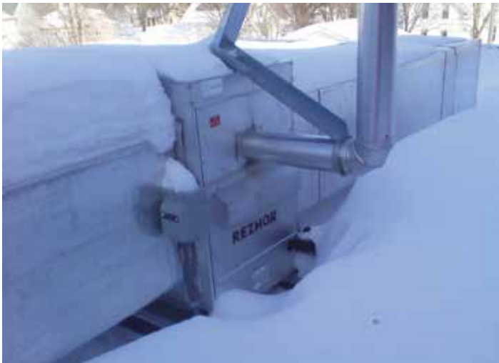
Reznor Rooftop Mounted Duct Furnace
